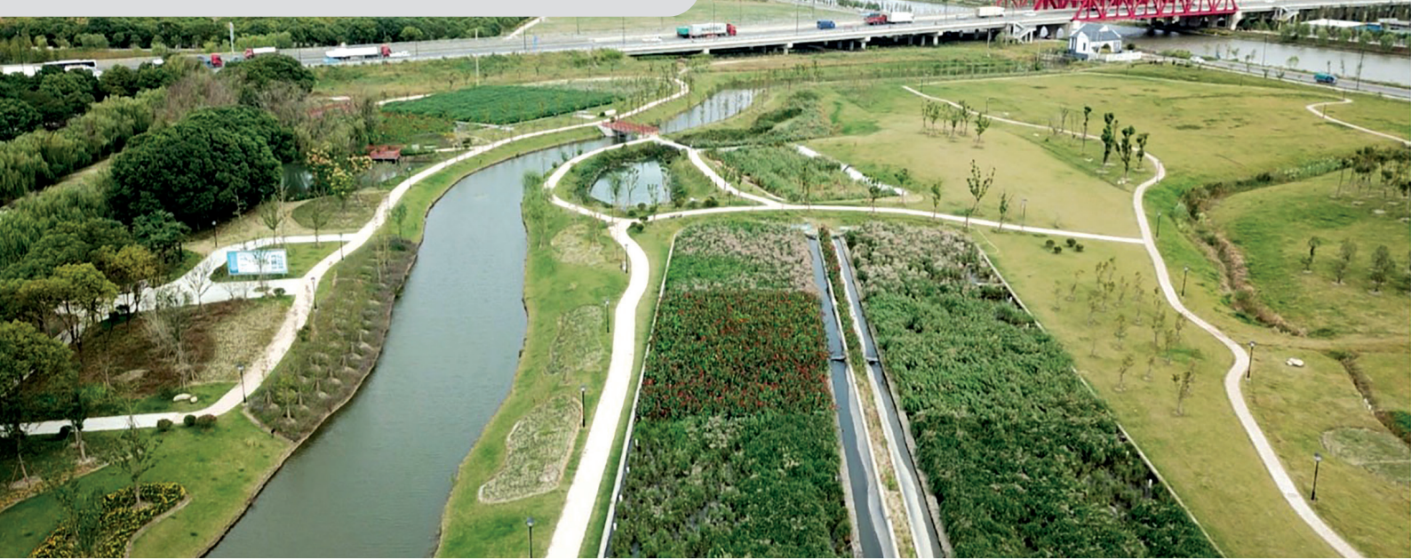
Figure 2 Hong Shuang Lou 3,000 m 2 demonstration wetland for CSO retention and filtration
